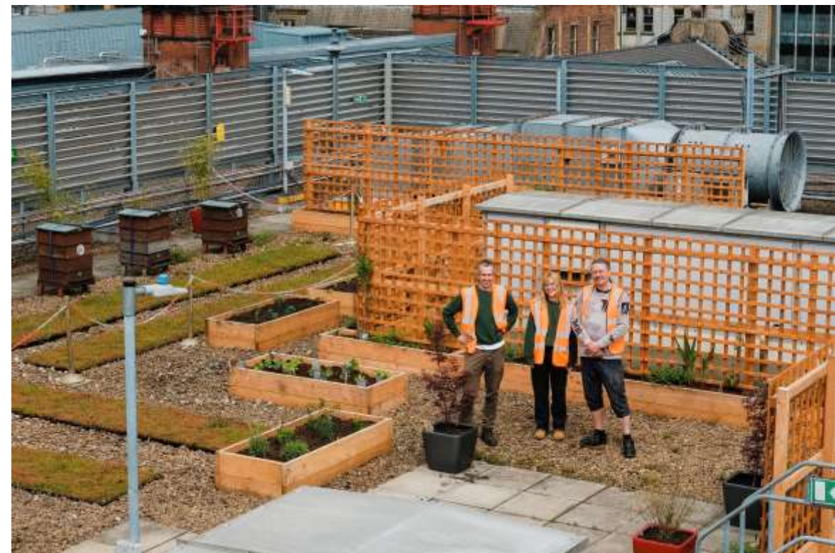
Printworks Green Roof. Client: Printworks Manchester
